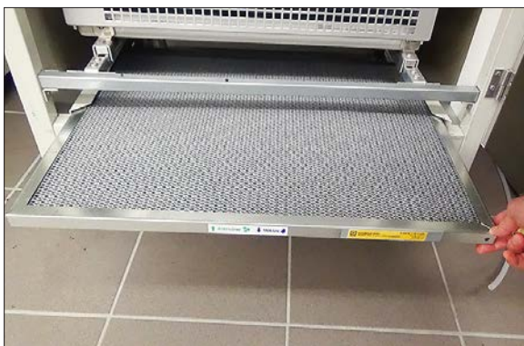
Figure 15.6d: Chiller air filter location.
